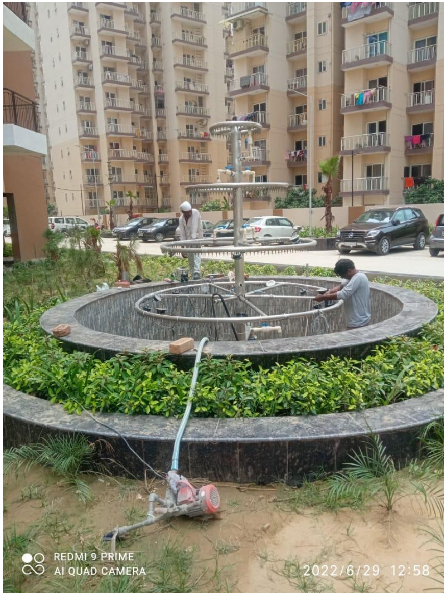
Fountain installation work in front of school is in progress
