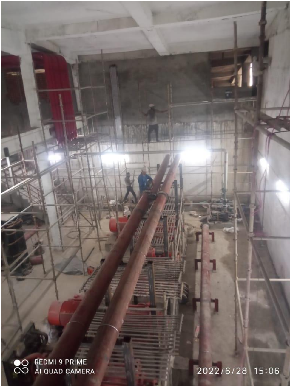
Pump Room: connection work is in progress.
