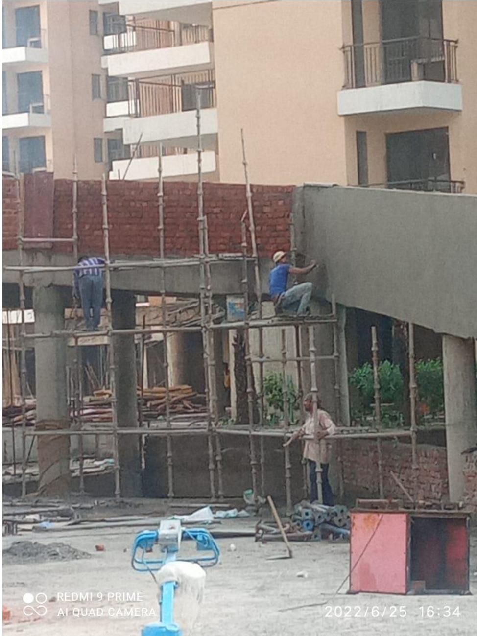
Ramp plaster work is in progress
