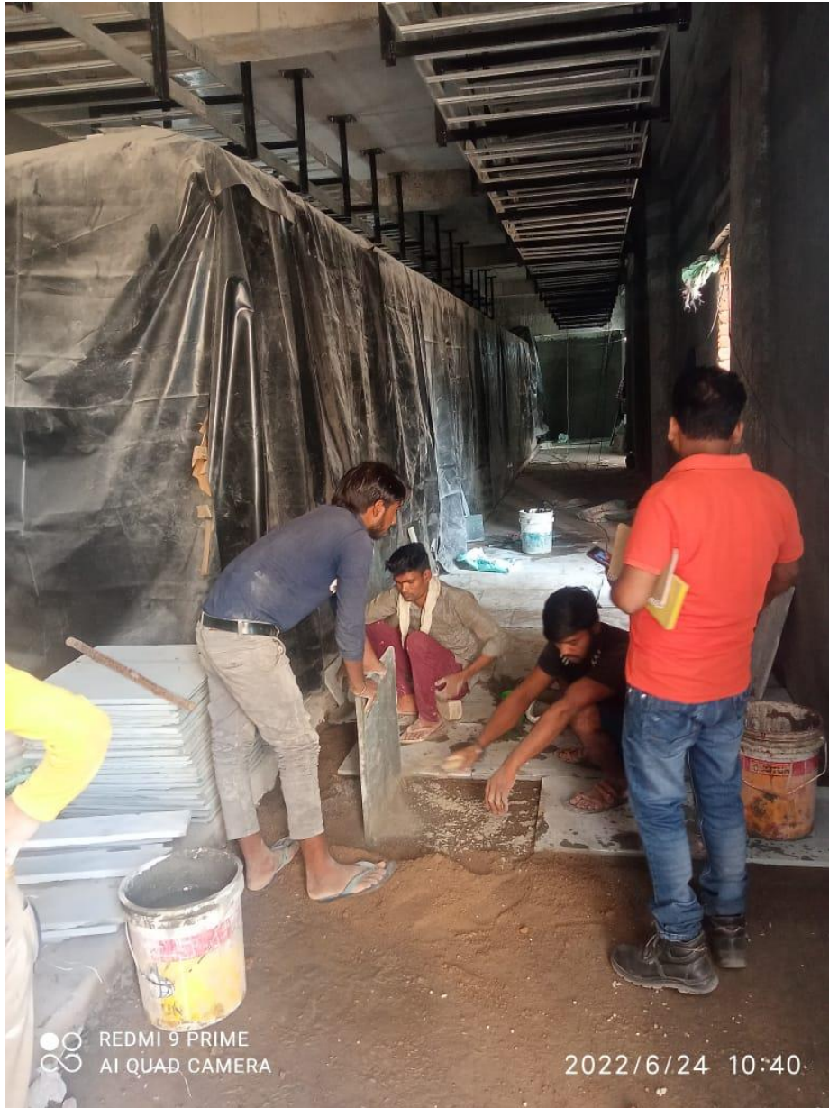
LT Room, Floor tiling work is in progress
