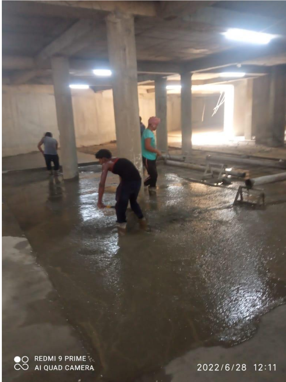
Tower E Basement Trimix work is in progress
