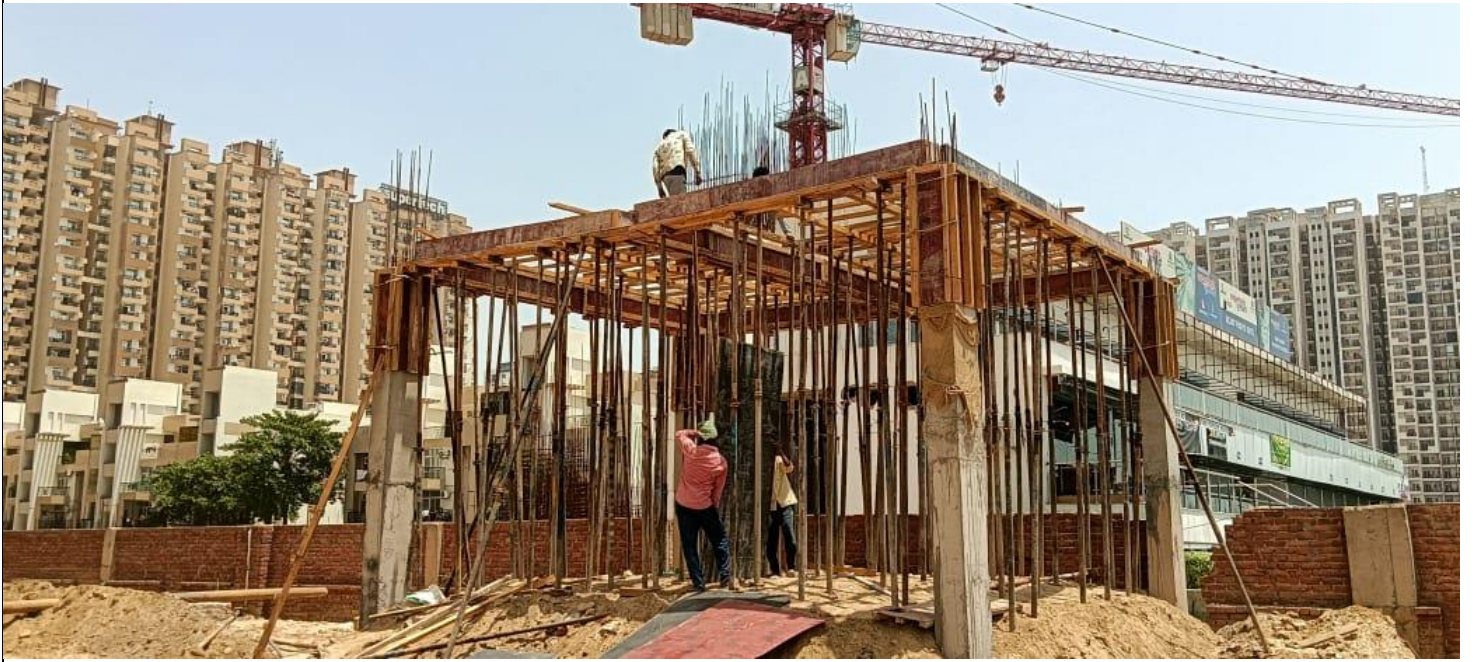
VCB Room construction work is in progress
