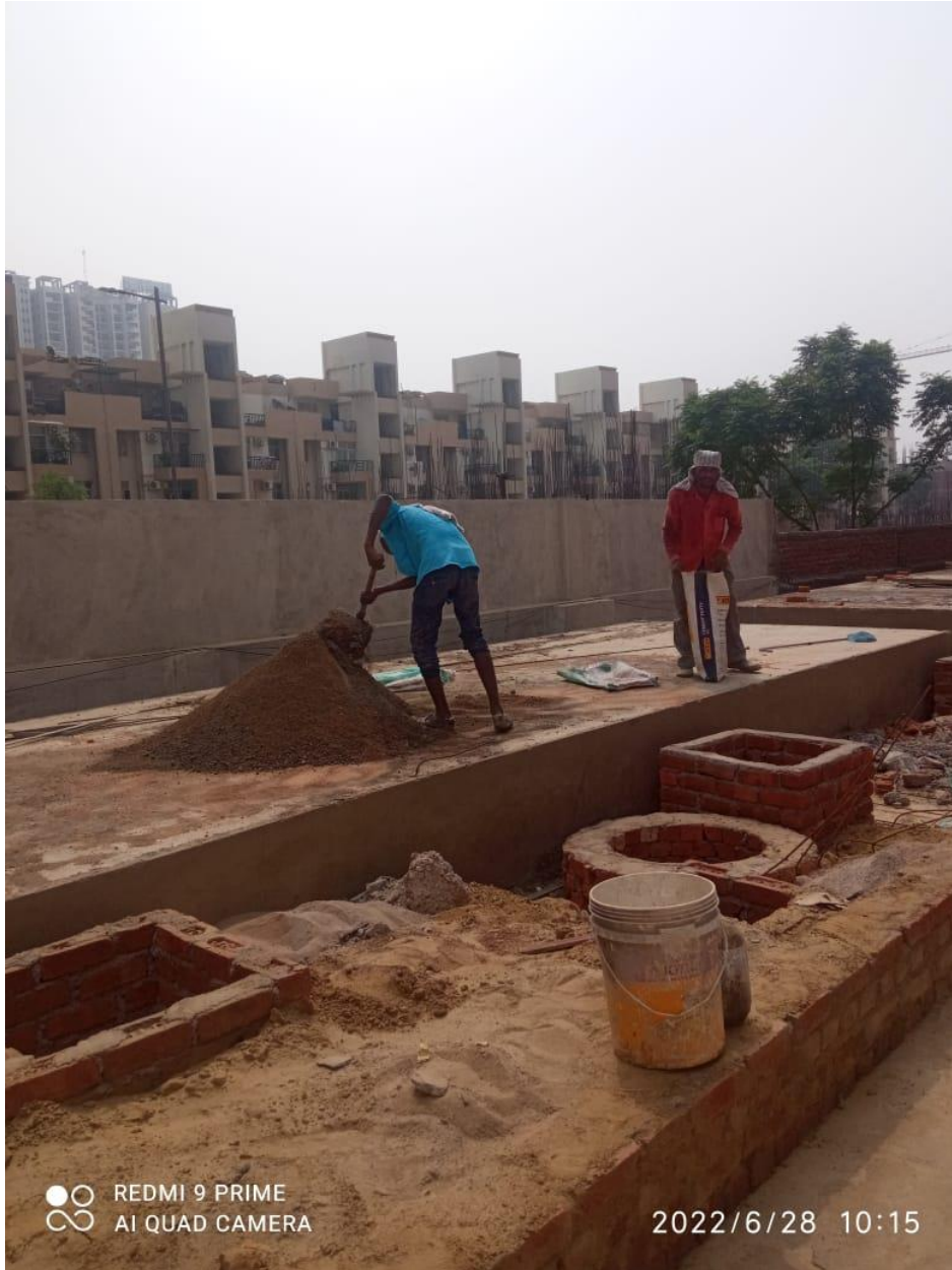
Near Tower D, E : Chamber brickwork is in progress
