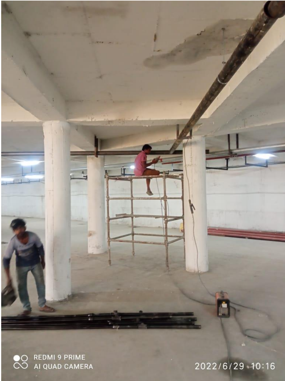
Fire hydrant installation work in basement is in progress.
